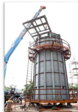
Hot Oil Heater
