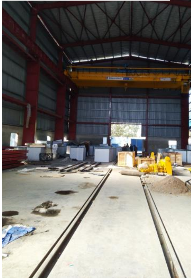
Clean room Shed Odhav
