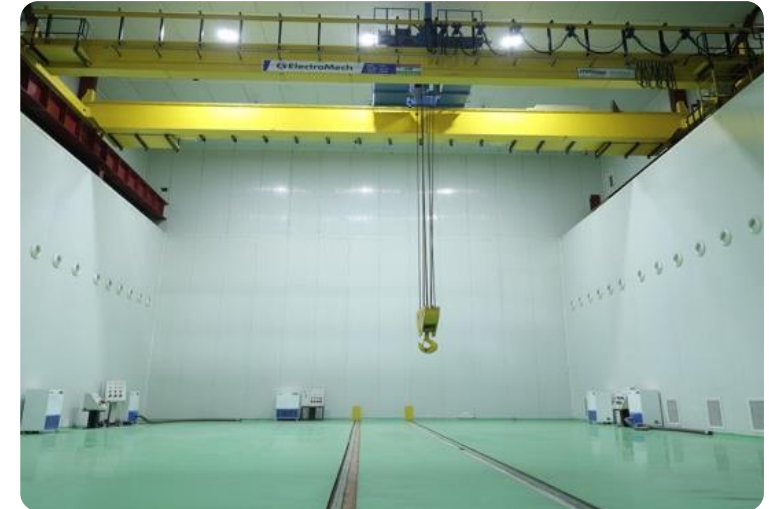
ISO 8 Class Clean Room for Exotic Material Fabrication (500 m 2 Area)
